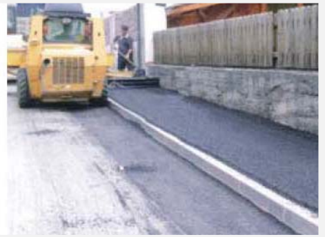
Laying sidewalk around gutter
